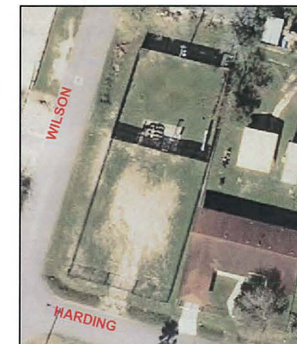
Lift Station No. 3 110 Wilson St. Laguna Heights
