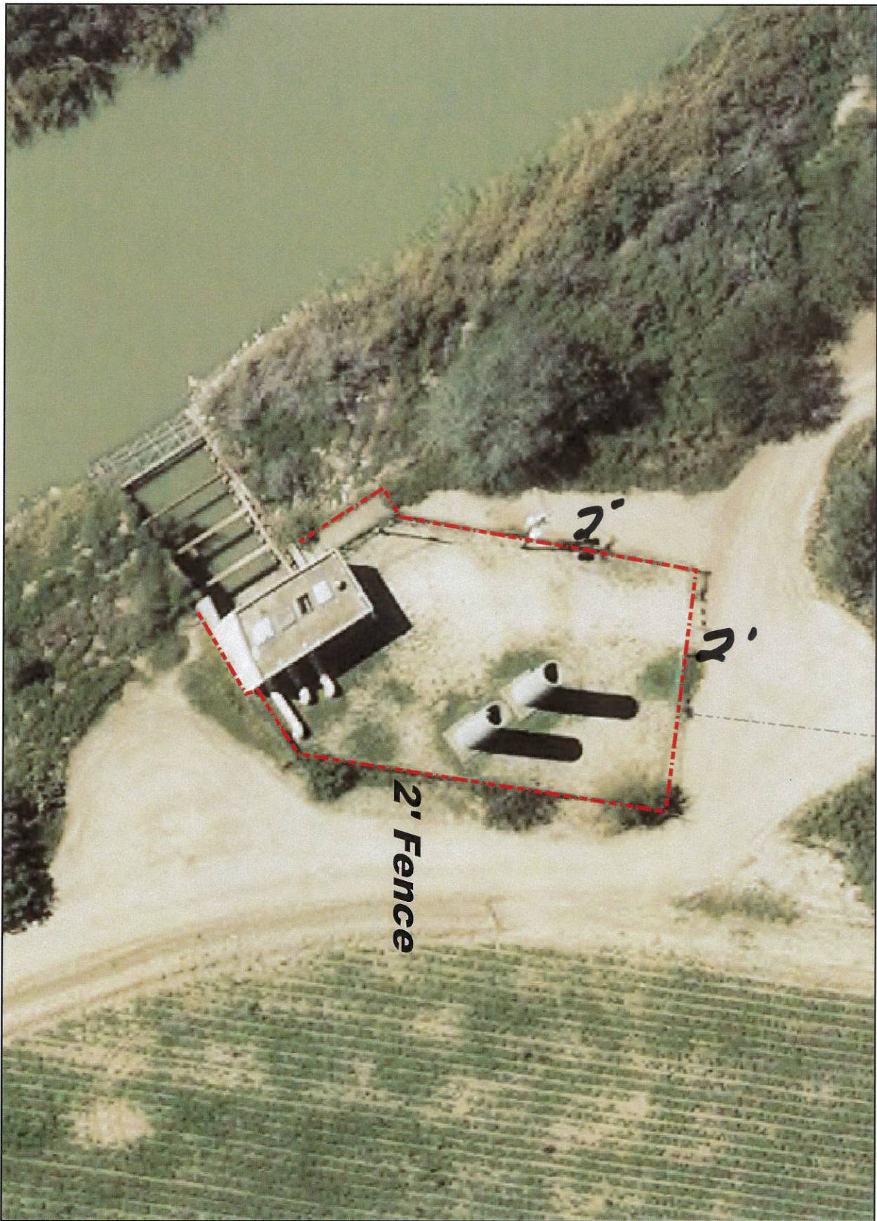
River Pump Station (Hurman Rodriguez Rd, El Ranchito Area)
