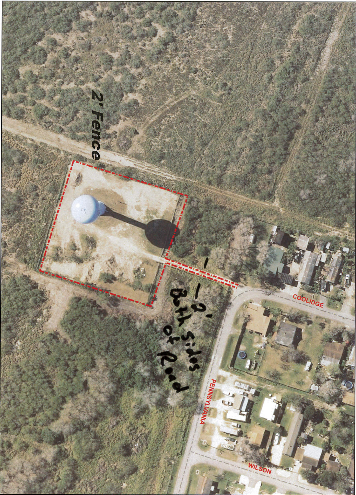
Elevated Water Storage Tank #5, Corner of Coolidge & Pennsylvania, Laguna Heights
